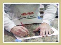
**Step 1** - **Templating:** - Reduce the paper template provided by sink manufacturer by 5/16" to create a new template. Reducing the template allows clearance for the drop-in sink. Fasten template to the stone using small pieces of tape, then trace.
