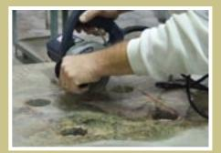
**Step 3 - Cutting:** - Install the Alpha® Eclispe II blade on the Alpha®AWS-125WetStoneCutter. Slowly plunge the blade into the cut line of the sink hole. Don't push it all the way through, step cutting is highly recommended. (Step-cutting requires 2 passes to complete).
