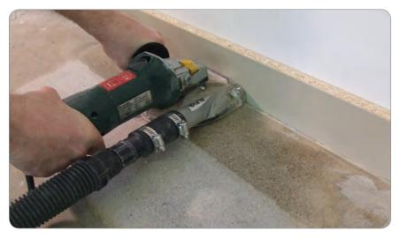
Alpha<sup>®</sup> introduces the universal concrete surface polishing system for concrete contractors who work on decorative surfaces. This system creates a superior surface polish on concrete whether you are using them wet or dry and by high or low rpms. The WDC Series is available in grits of 60, 150, 300, 500, 1000, 2000 & 3000. Thanks to the patented Alpha<sup>®</sup> Variable Drive System, you can polish using any polisher, or high-speed angle
