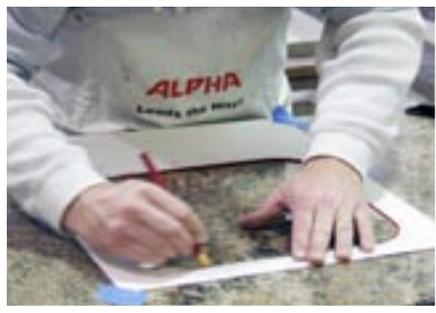
**Step 1 - Templating:** - Reduce the paper template provided by sink manufacturer by 5/16" to create a new template. Reducing the template allows clearance for the drop-in sink. Fasten template to the stone using small pieces of tape, then trace.
