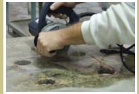
**Step 3 - Cutting:** - Install the Alpha® Eclipse II blade on the Alpha® AWS-125 Wet Stone Cutter. Slowly plunge the blade into the cut line of the sink hole. Don't push it all the way through, step cutting is highly recommended. (Step-cutting requires 2 passes to complete).
