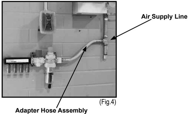
**NOTE:** Adapter Hose Assembly is only available for Part No. 1030-0022 (53CFM) and 1030-0023 (106CFM) F/R Manifolds.
