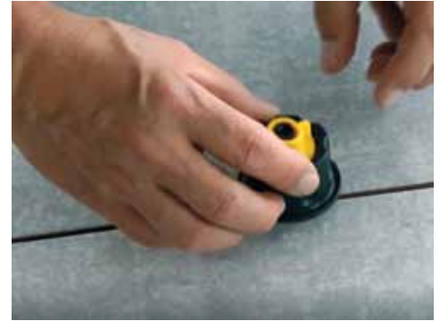
4. Turn Black Base to Tighten
